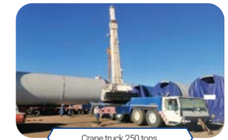
Crane truck 250 tons
