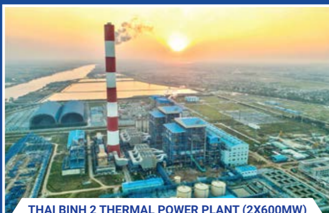
THAI BINH 2 THERMAL POWER PLANT (2X600MW) Thermal Power Street, Xuan Hoa, Thai Thuy, Thai Binh
