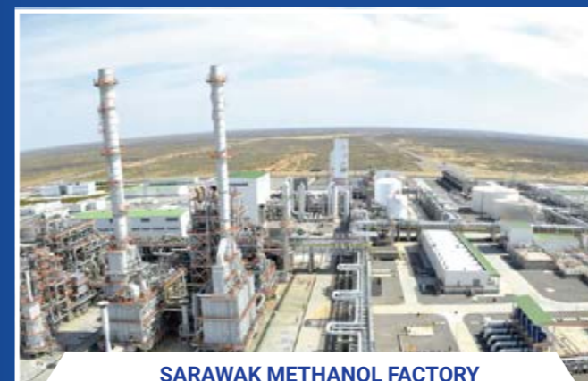
SARAWAK METHANOL FACTORY MALAYSIA (5,000 tons/day)
